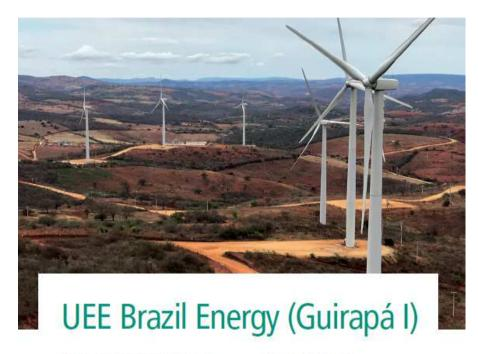
BW Guirapá I is a 170.2 MW wind generation facility located at Pindaí and Caetité, Bahia state. It is composed of seven wind farms with 92 wind turbines in total and produces enough electricity to power up approximately 366,000 households.
